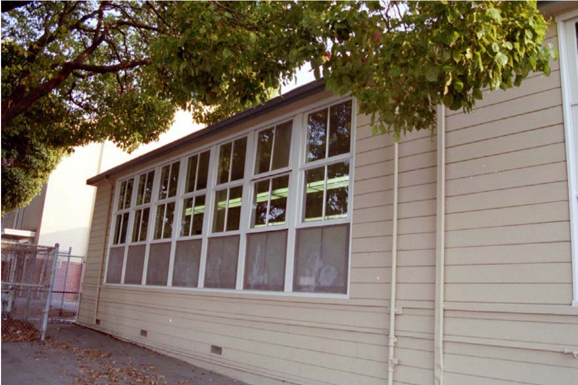
Figure 10: Additional Classroom Building 1 north face
