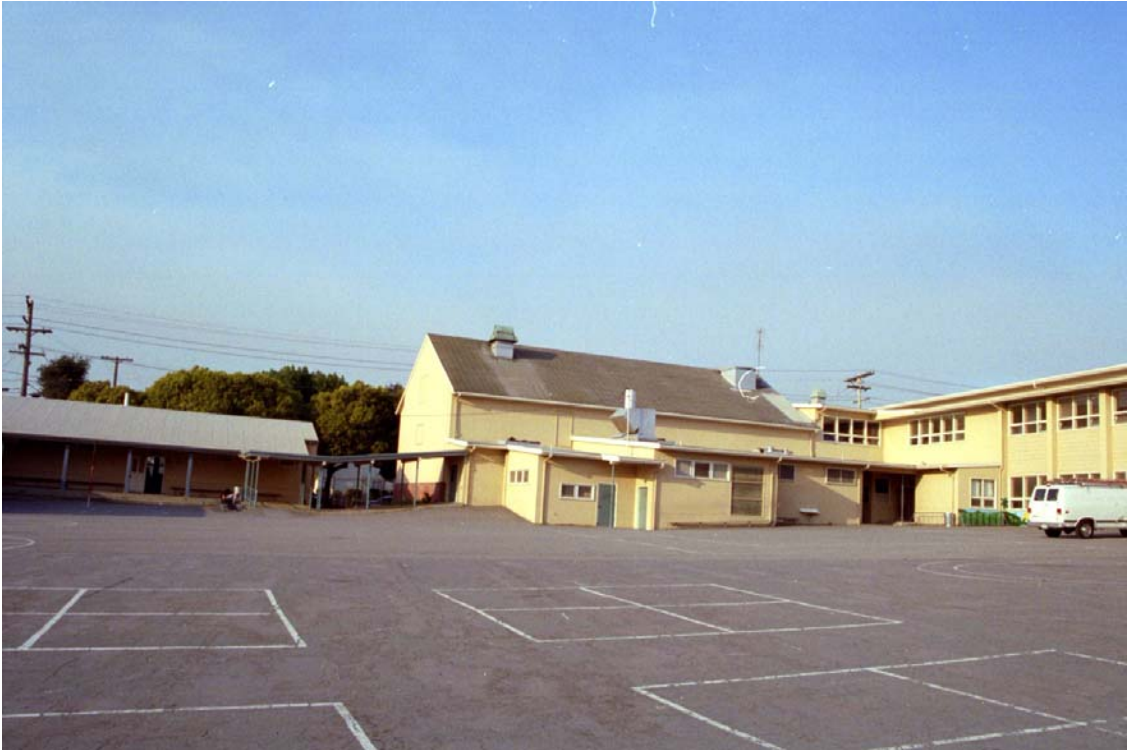
Figure 6: Auditorium Building south face
