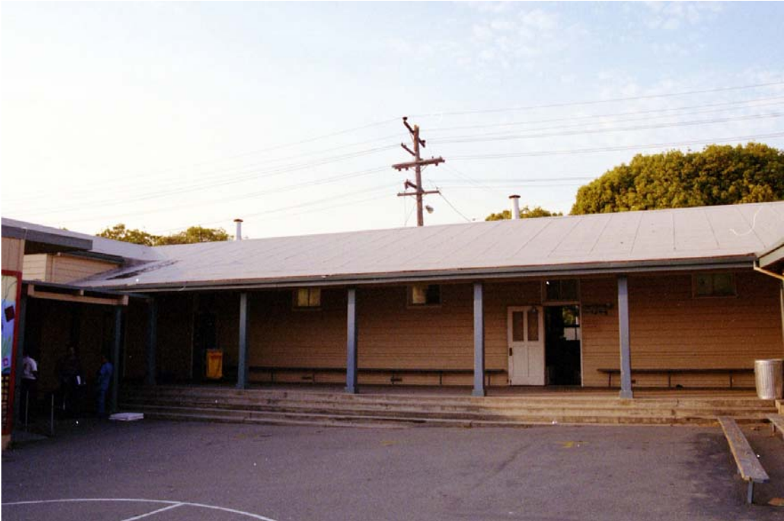
Figure 8: Additional Classroom Building 1 south face
