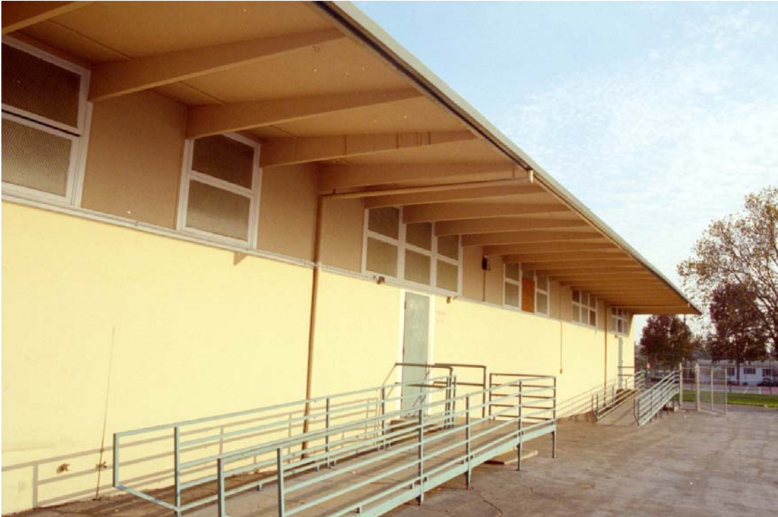
Figure 5: Cafeteria Building east face
