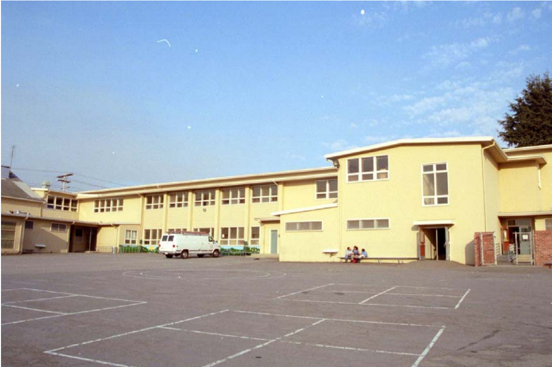
Figure 7: Main Classroom Building east face
