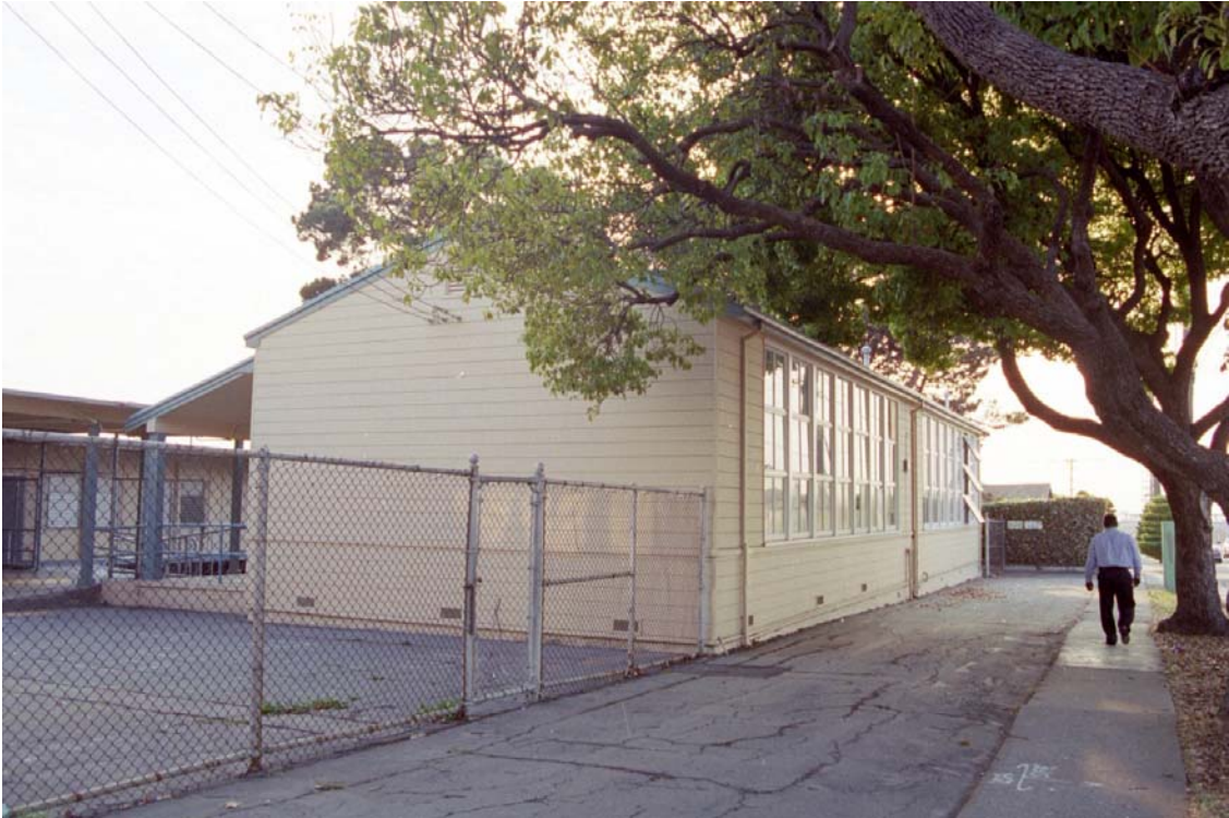
Figure 11: Additional Classroom Building 2 north face
