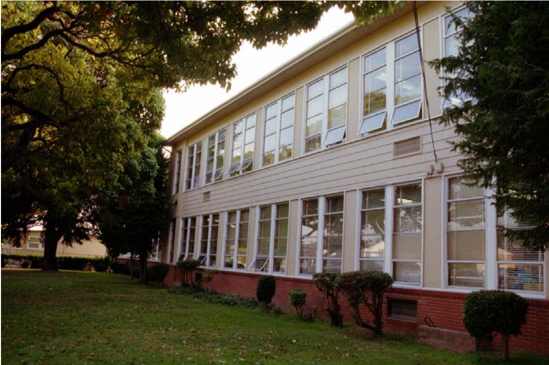
Figure 4: Main Classroom Building facing Ashbury Avenue
